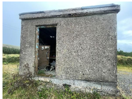
Plate 4-8 Brick building access.
