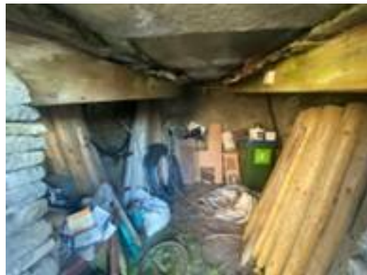
Plate 4-6 Stone shed interior
