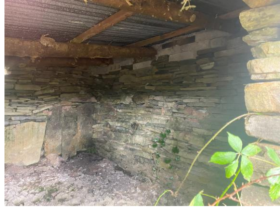
Plate 4-2 Stone structure interior
